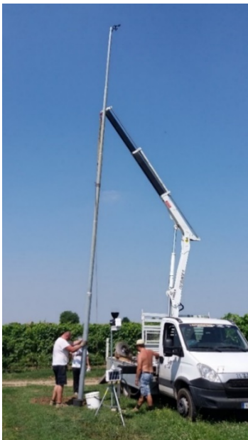
Fig. 10a Installation of the anemometer pole.
